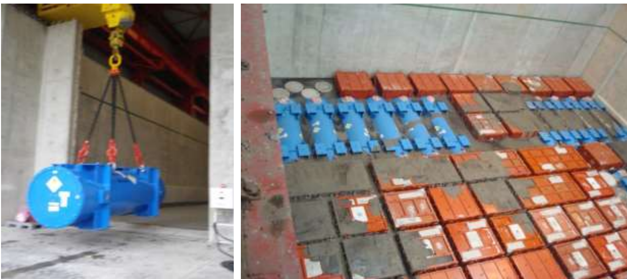
Fig. 2 Disposal of Non-standard Waste Package in Disposal Vaults at Centre de l'Aube
